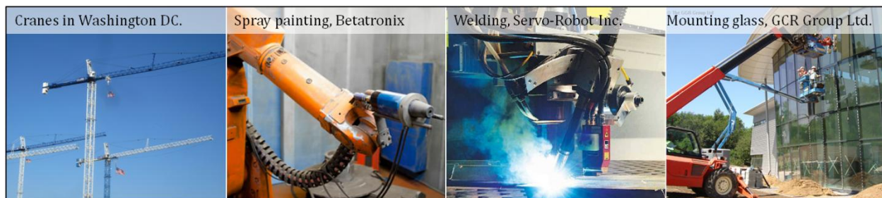
Figure 2.1.a. Sample of robot aided construction tasks in industry today.
